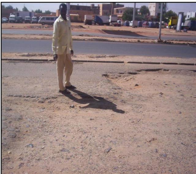
Plate (1): Severe distresses of potholes and rutting appear on Alazhari Road surface
