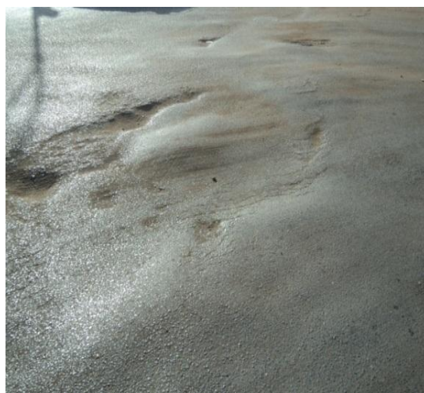
Plate2. Severe distresses of potholes and heave exist on Alarda Road surface
