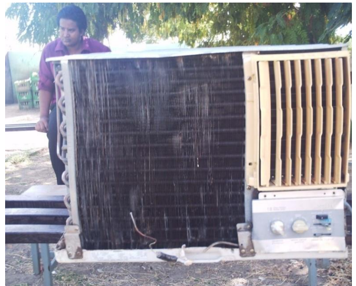
Fig.2. Evaporator coil after cleaning
