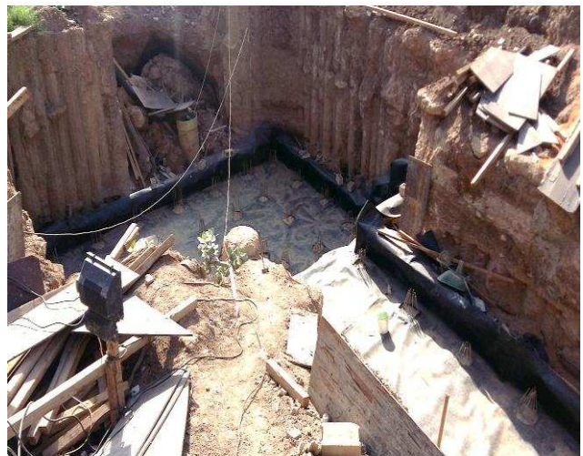
Fig. 8. Falling down of excavation sides after dewatering
