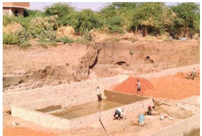
Fig. 11. Sliding failure of the excavation sides created large cavities
