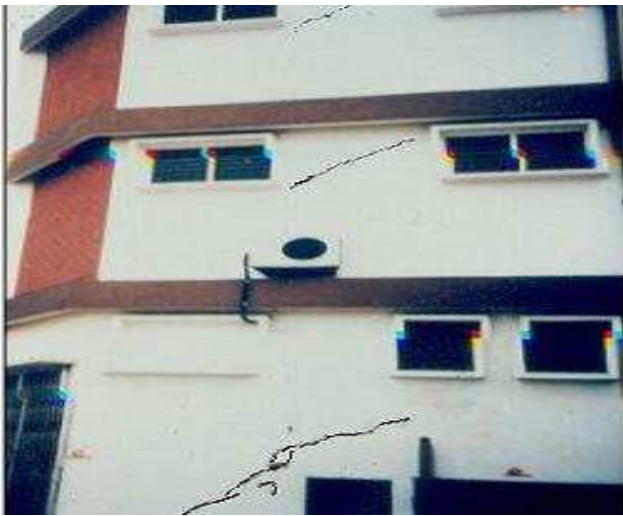
Fig. 5. Severe cracks in the external walls of a house, [14]
