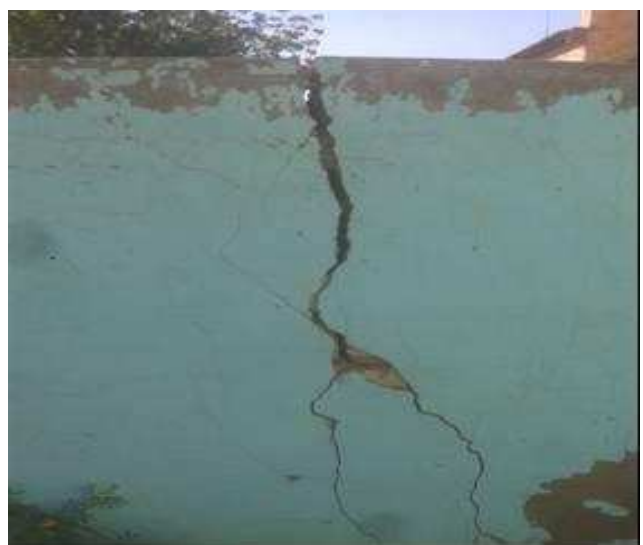
Fig. 9. Serious cracks in walls of adjacent buildings
