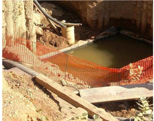
Fig. 7. Water filling the site and erode the excavation sides.
