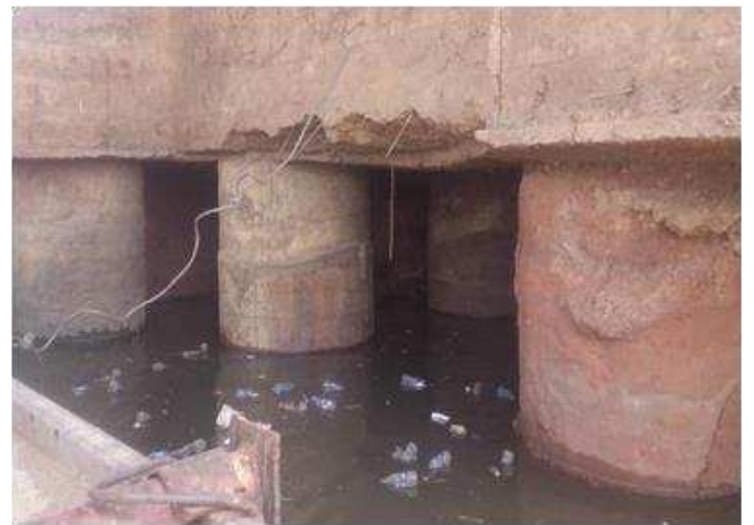
Fig 6: The foundation piles surrounded by water
