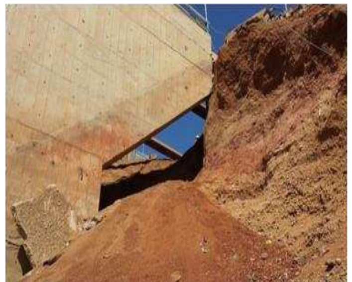
Fig 7: Embankment soil escaped away from the approach slab
