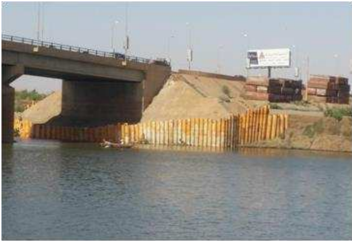
Fig 8: Sheet pile installed around the abutment
