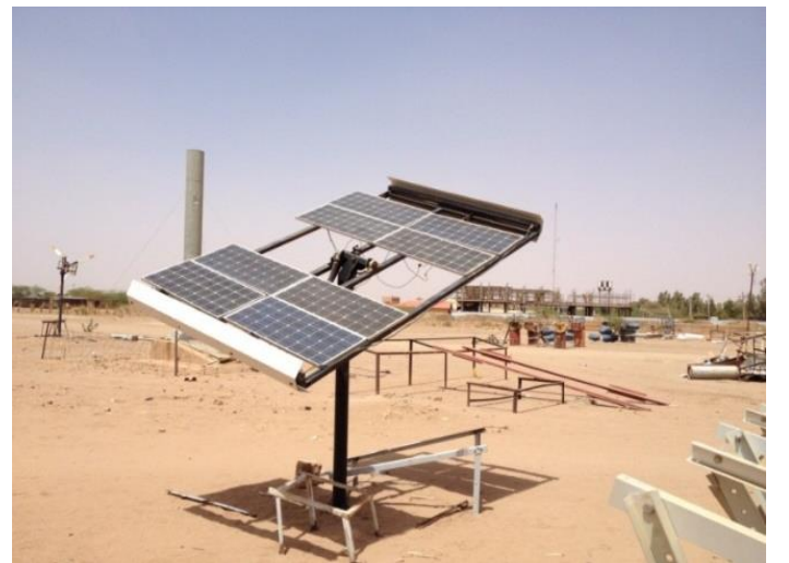
Fig. 1. Solar Tracker with Photovoltaic Modules
