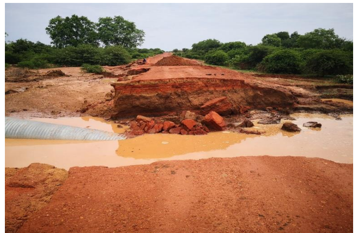
Fig .9. Erosion of soil due to pipe culvert failure in BNA road
