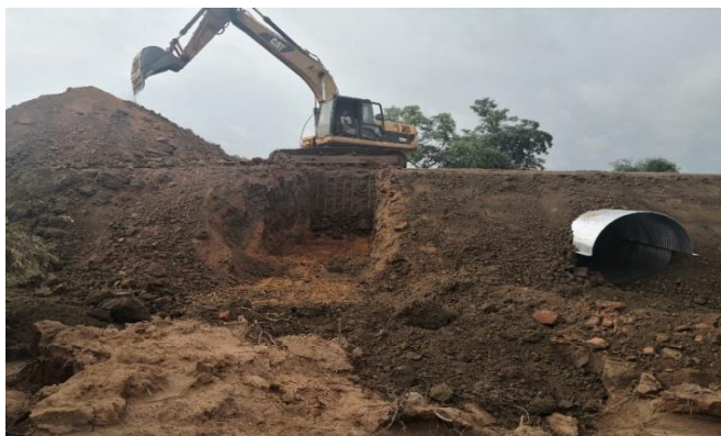
Fig .7. Pipe culvert installation in BNA road
