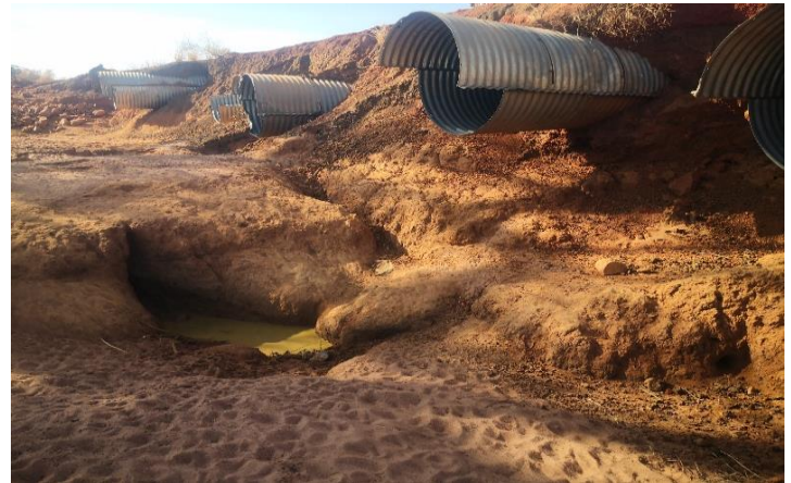
Fig .8. Erosion in the outlet in Sabreen
