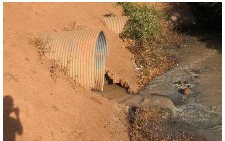
Fig 10: Erosion in protected pipe culvert in HTL road
