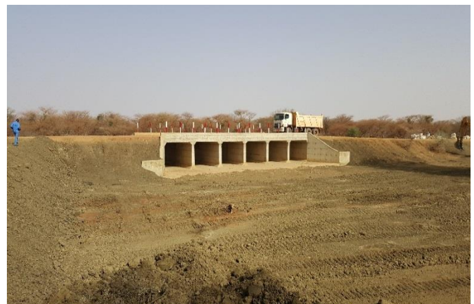
Fig.22. 6 cells concrete box culvert in HC pipeline road
