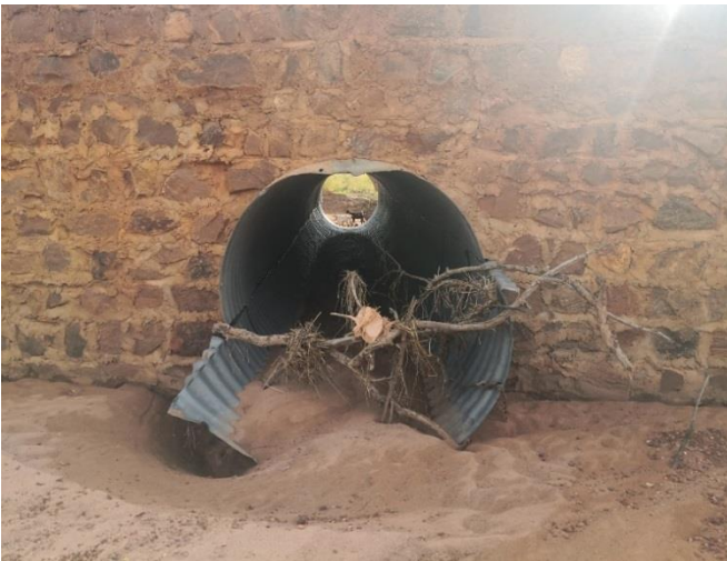
Fig. 4. Floating tree in pipe culvert inlet in Sabreen
