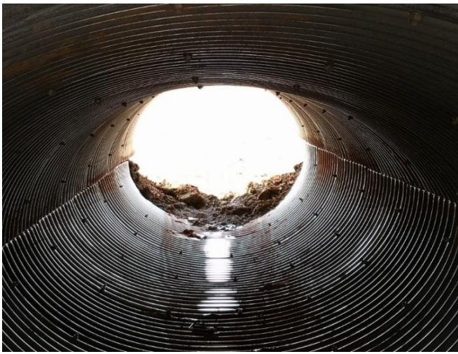
Fig .3. Deformation in pipe culvert in Shag Yahia
