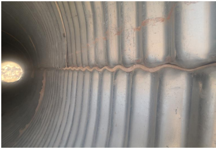
Fig. 11. Rubber sheets sandwiched in pipe culvert in BV#2 KP7.
