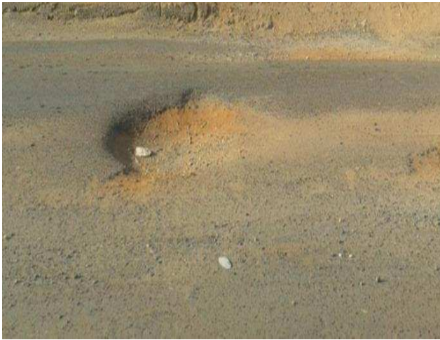
Fig. 4: damaged surface with large potholes on road R1
