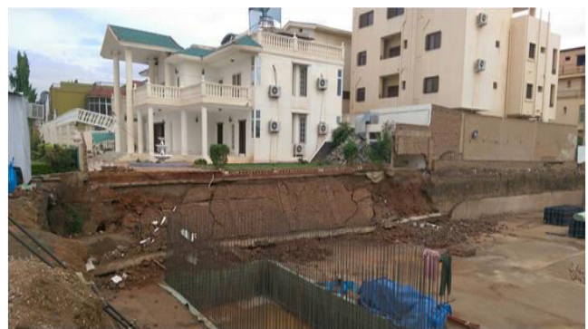
Fig. 9 The Shoring Piles Distributed All Around
