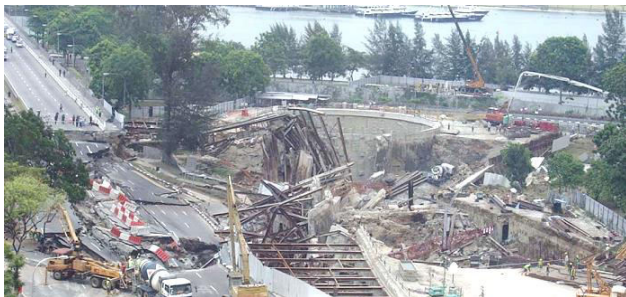
Fig. 4 Collapse of Nicoll Highway at MRT Station in Singapore, [7]
