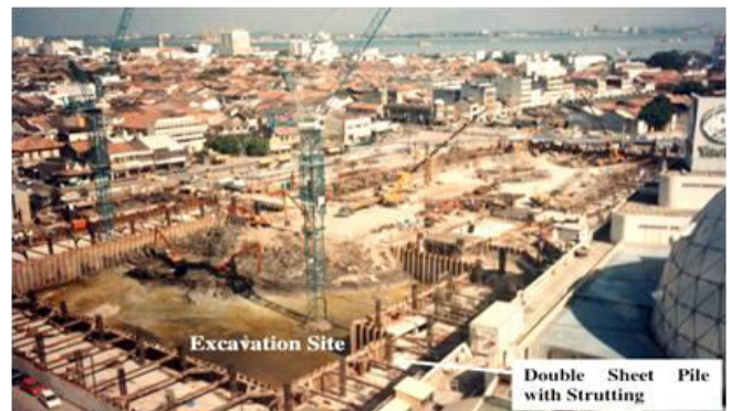
Fig. 5 The Site Condition of Penang upon Reaching the Final Excavation Level [8]
