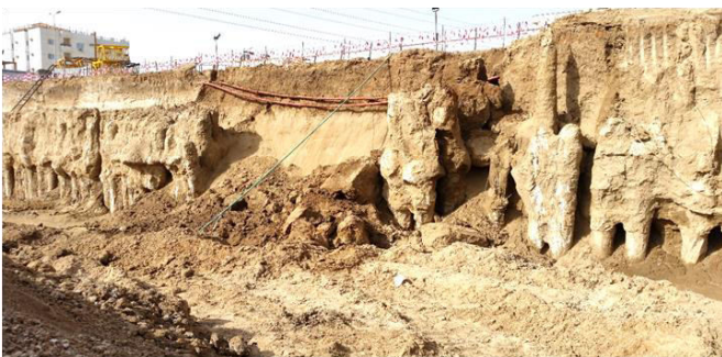
Fig. 7 The shoring piles distributed all around the perimeter of the building basement
