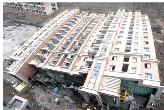
Fig. 2 Building Collapsed in Shanghai, [6]
